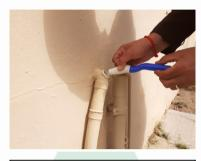
Step 5— While holding the fold in place, insert the WUNNEL into the inspection eye. It should expand to its shape at rest.
