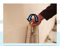
Step 2— Remove cover by turning it anti-clockwise (Store in a safe place for future re-attachment)
